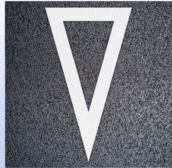
Give Way Road marking
